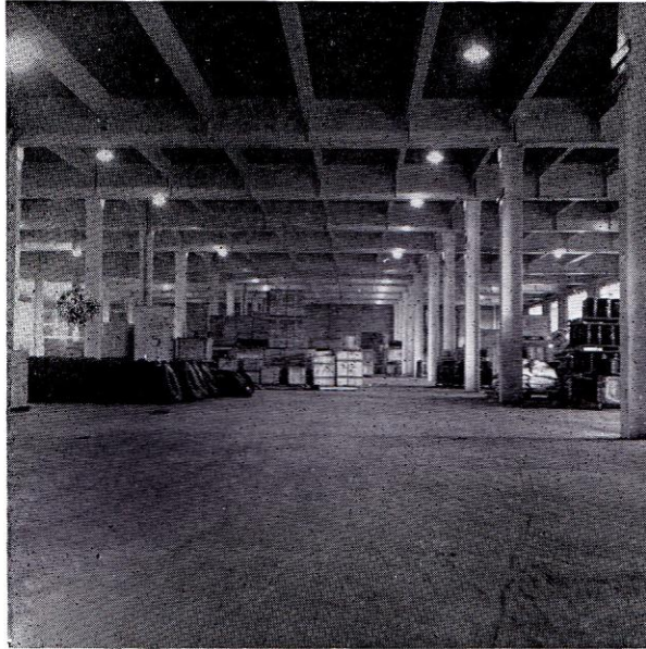
Interior of New Warehouse
